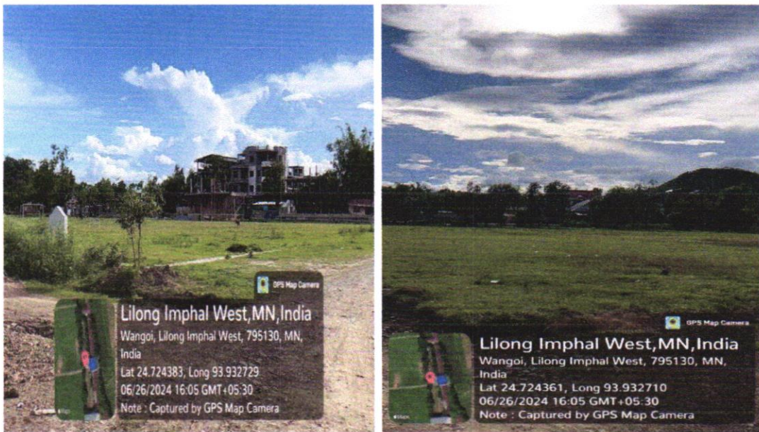
Fig 11: Football field with open gallery at the College entrance
